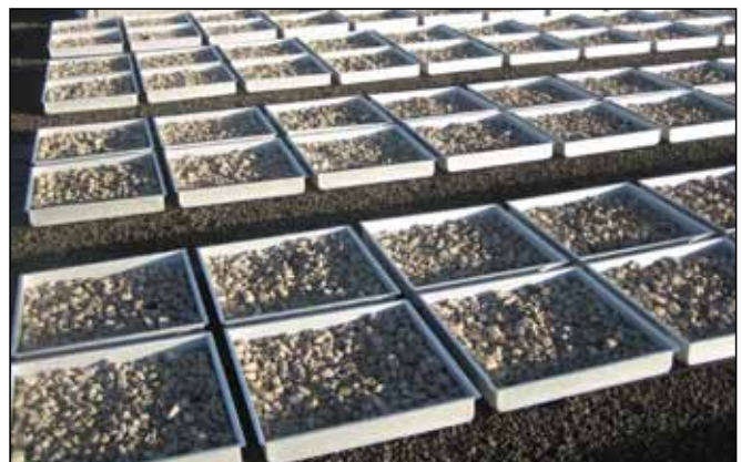
DEP installed a tray and ballast system in the fourth quadrant that detains stormwater in 1,600 trays before it eventually drains off the roof.
