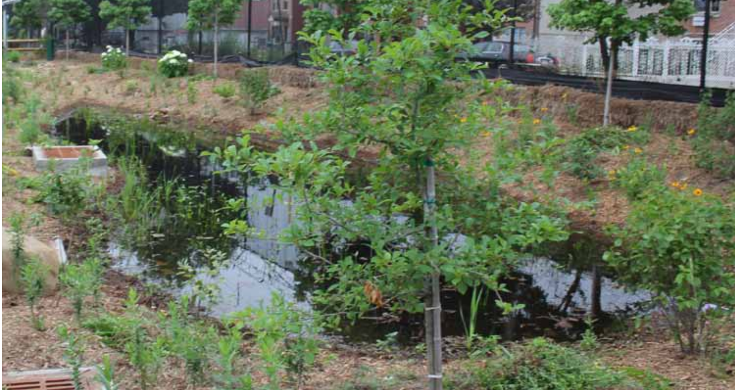
In May 2011, DEP constructed a pilot mini-wetland and bioswale system in the parking lot of an MTA bus depot in Brooklyn.
