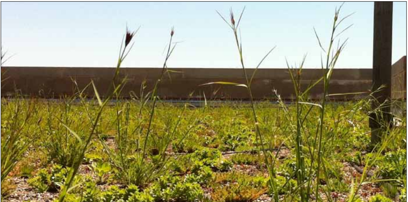
Green roofs are designed to absorb rainwater until it can evaporate or be consumed by the vegetation through evapotranspiration.
