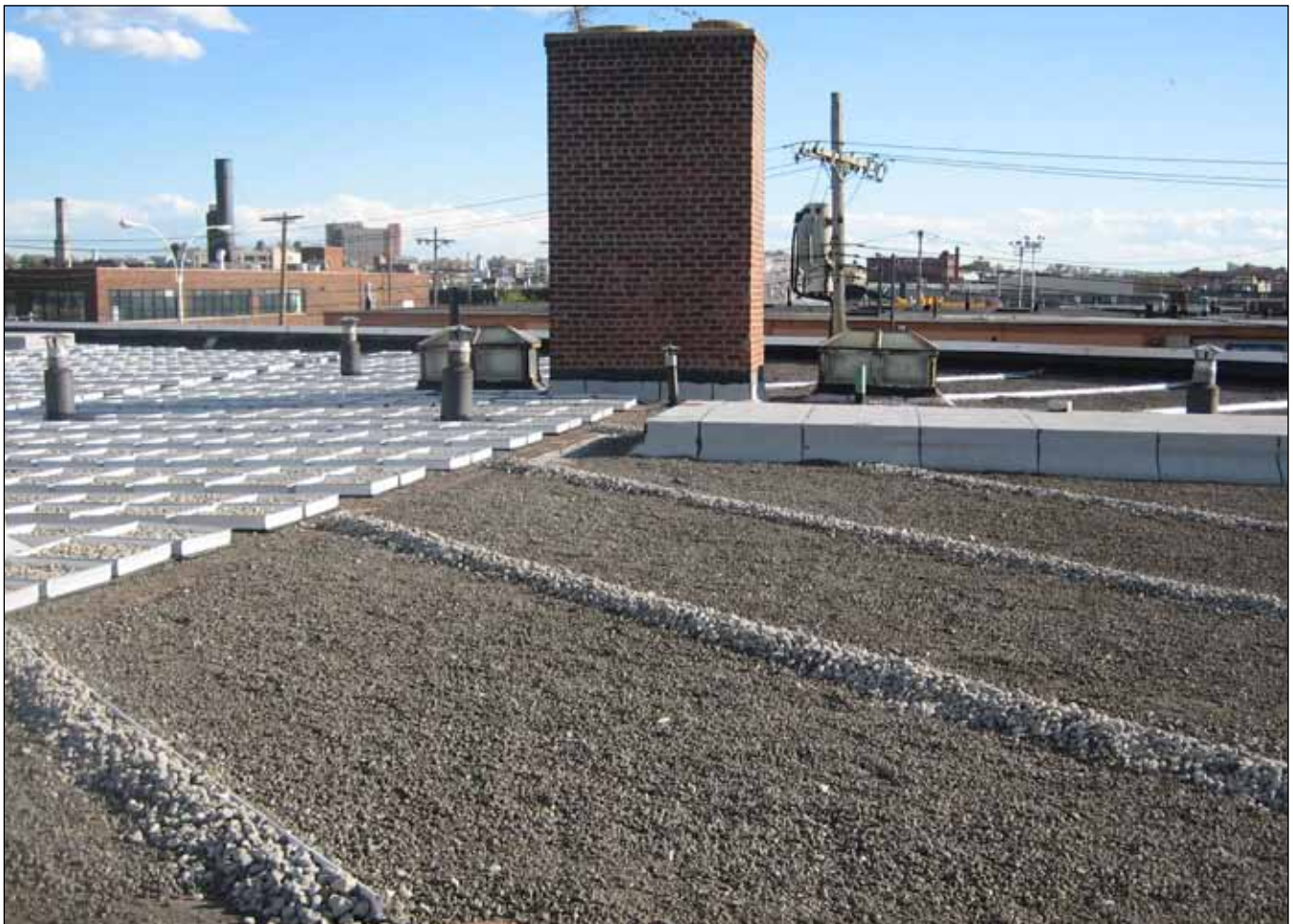
DEP piloted three different blue roof technologies on the rooftop of one of our general storehouse facilities in Brooklyn. The design includes a tray and ballast system, on the left side of the above image, and an intermediate check dams system, on the right side of the image.
