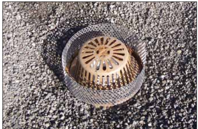
DEP installed a modified drain cover in the second quadrant to control the flow of stormwater off the roof.
