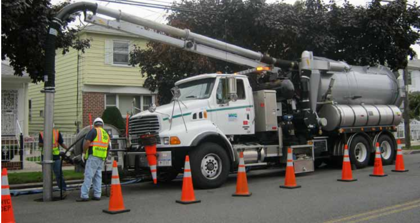
DEP uses Vector trucks to remove sedimentation from the sewer system, increasing its capacity to hold wastewater during wet weather.
