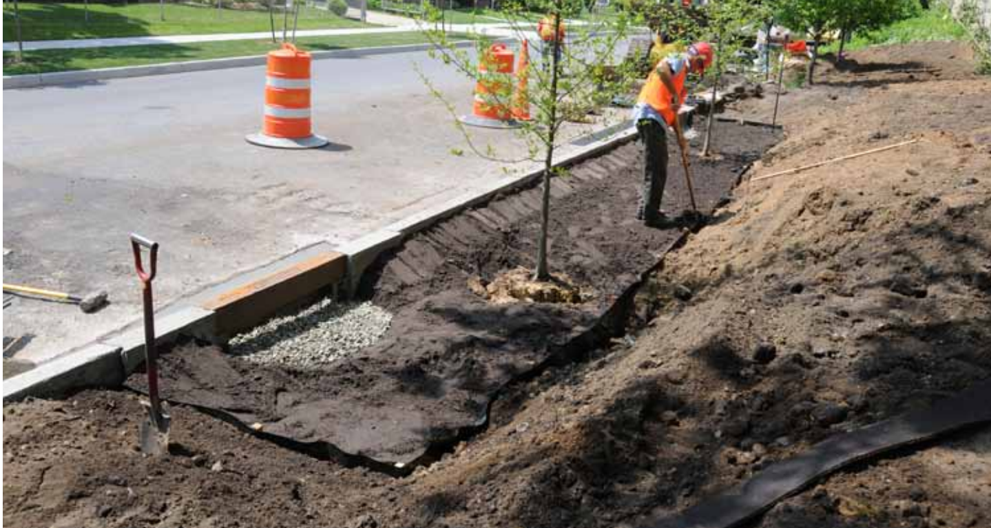
Streetside infiltration swales, such as this one located in Brooklyn, can manage thousands of gallons of stormwater each year.
