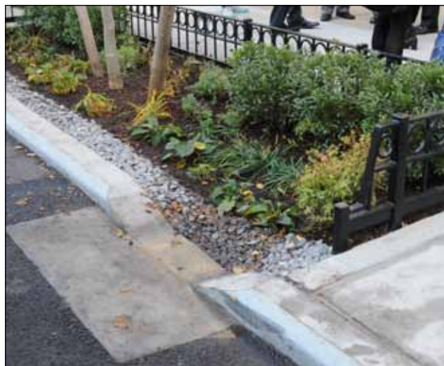
After evaluation of the first generation of inlets, DEP replaced some of the inlets with depressed curbs to increase stormwater conveyance into the ETP or SSIS.
