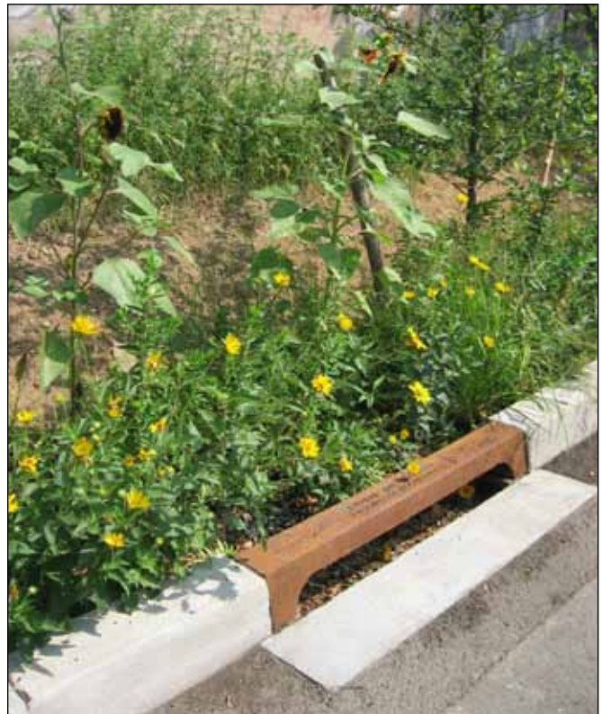
SSISs are 40 feet long, five feet wide, and 4.5 feet deep, and have only one subsurface layer made of engineered soil.
