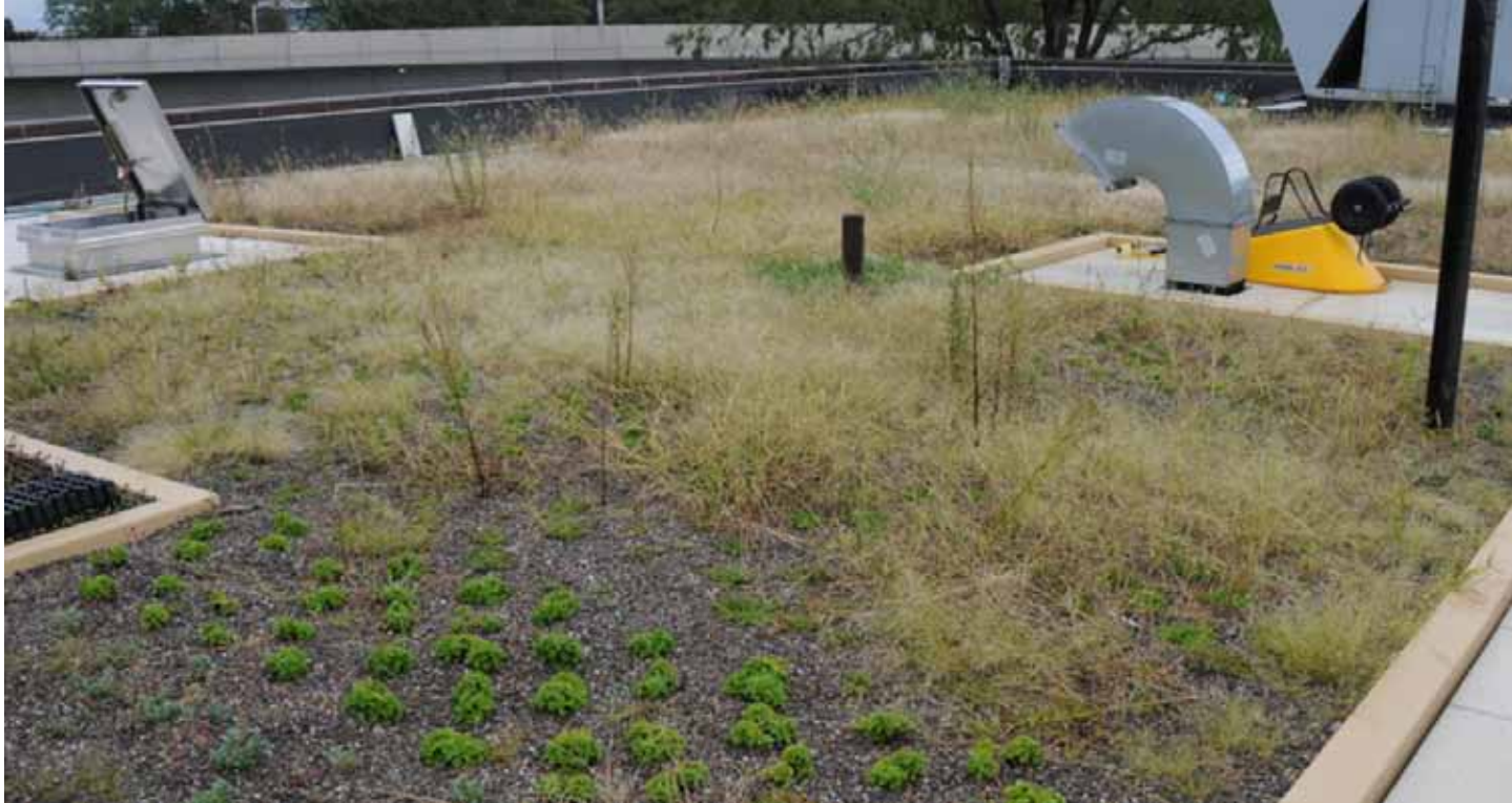
The Jamaica Wastewater Treatment Plant green roof manages more than 13,000 gallons of stormwater each year, reduces the building's absorption of ultraviolet light, and improves insulation.
